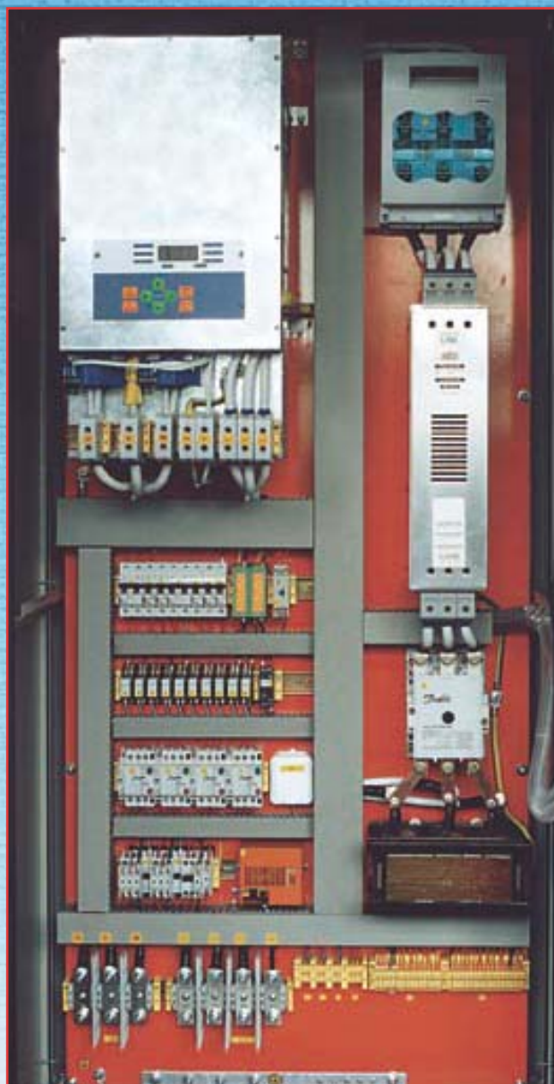
Speed regulation system of 90kW / 380V motor.
